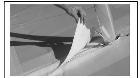
**Figure 7 Section 4. Install Pull Back Cover**
